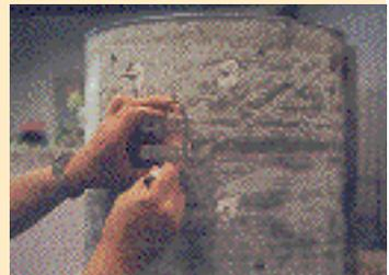
6. Mark the location for the terminal blocks. Drill and bolt them to the casing.
