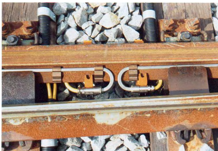
Stock rail heating in a vignole-rail point assembled with connecting head fasteners
