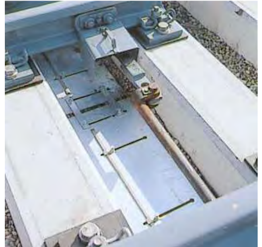
Point interlocking heating system on concrete sleepers
