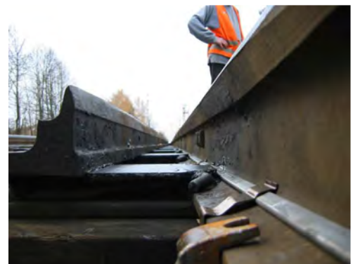
Position of heating element in free space between sliding seats and rail web
