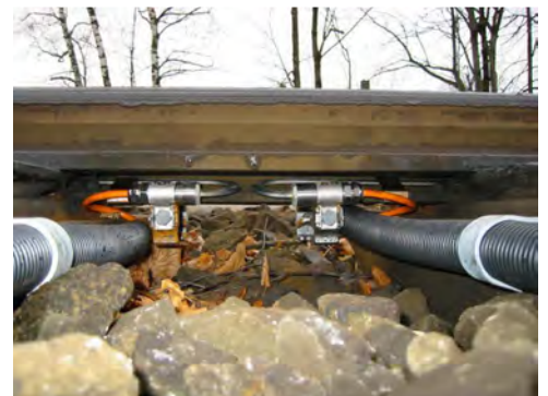
Switch blade gliding over connecting head; bottom view
