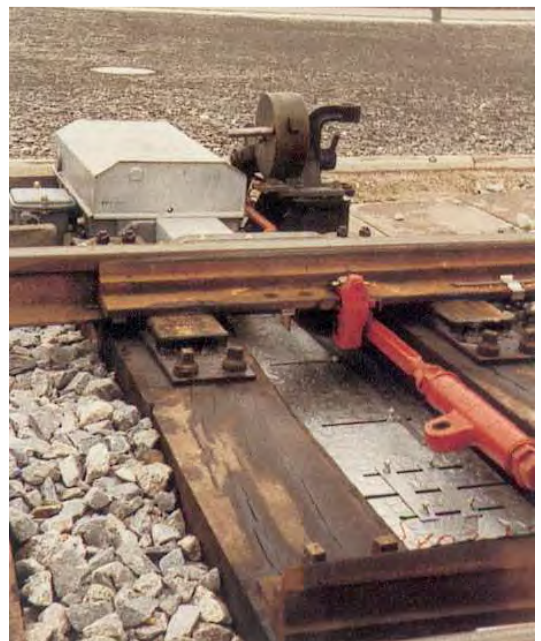
Point interlocking heating system placed underneath the switch rodding and embedded on ballast
