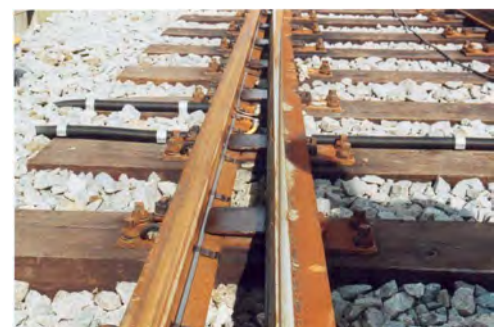
Switch blade gliding over connecting head; bottom view
