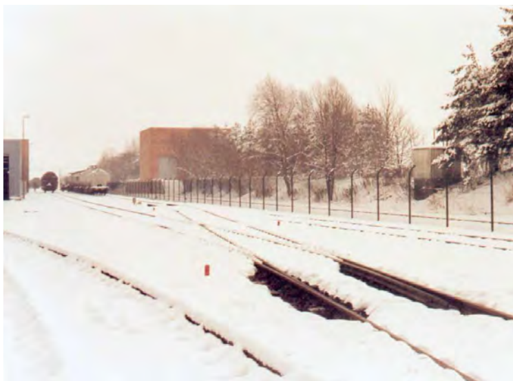
Switch blade heating and point interlocking heating system at wooden sleepers
