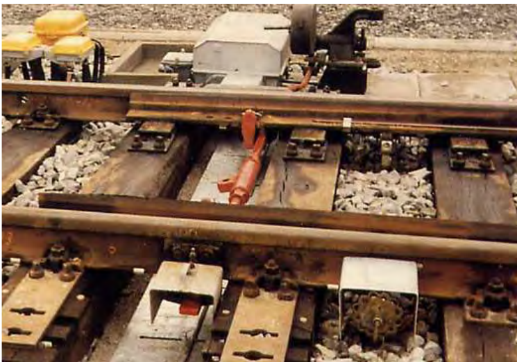
Switch blade heating and point interlocking heating system at wooden sleepers
