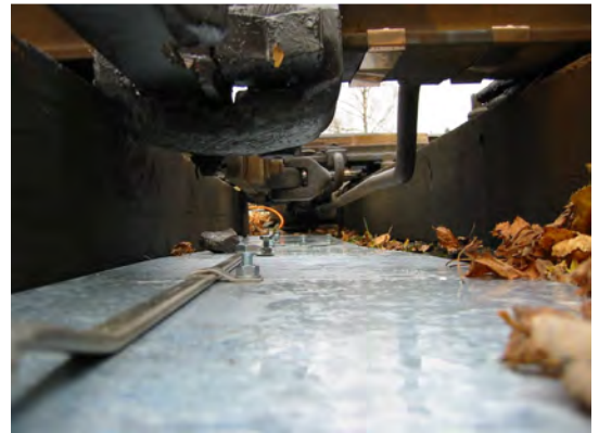
Point interlocking heating system placed underneath the switch rodding and embedded on ballast
